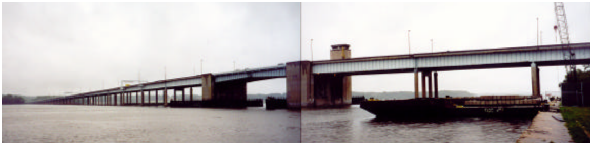
Existing Woodrow Wilson Memorial Bridge
