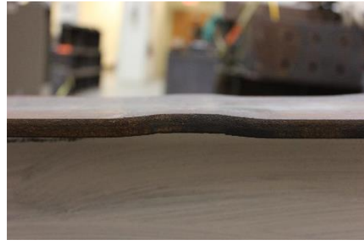
Bent steel flange in beam 3-M20-3C-RL
