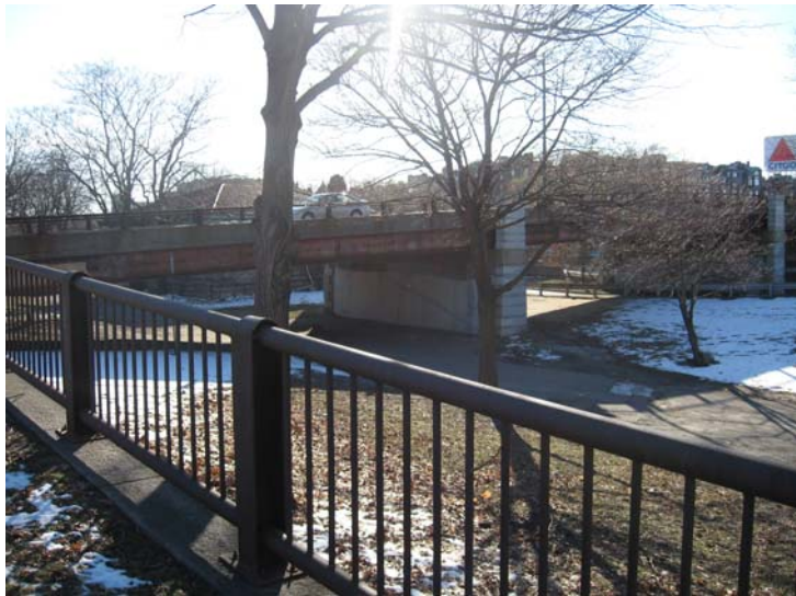
Figure 7.2C: Existing Retaining Wall
