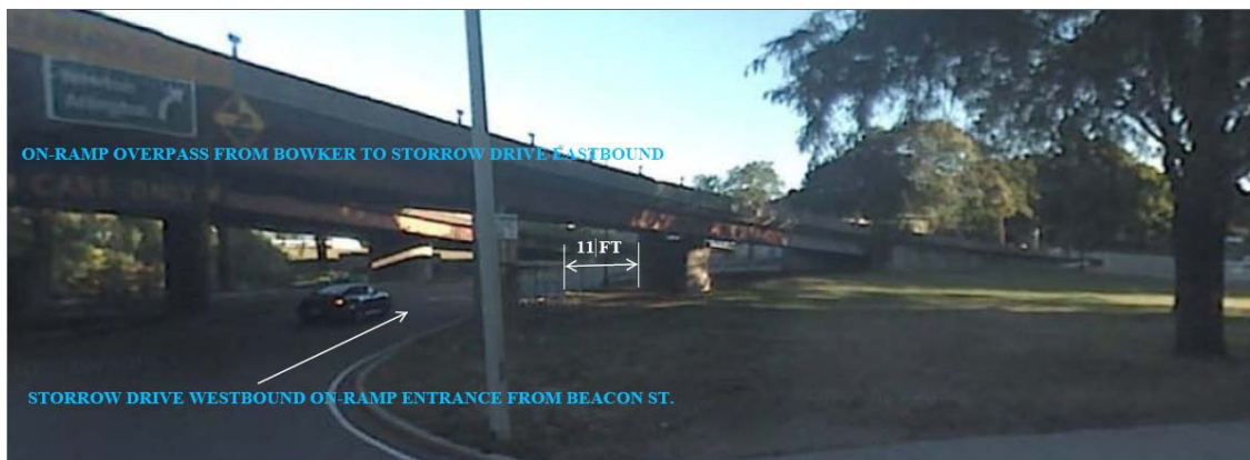
Figure 6.1C: Looking Northward from Beacon Street at the Storrow Drive Eastbound On-ramp Overpass from the Bowker Overpass and the Storrow Drive Westbound On-ramp Entrance from Beacon Street
